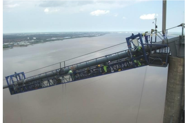
Gantry at tower top
