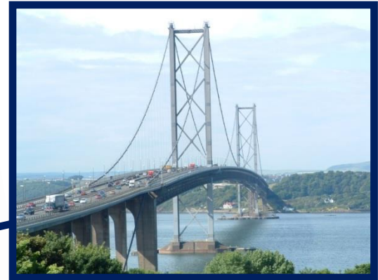
Forth Road Bridge
