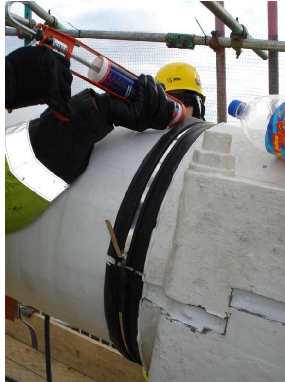
Install wedge & seal
